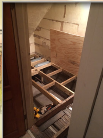
INSTALLED NEW STRUCTURE AND SUBFLOOR
