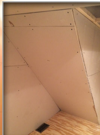
FRAMED SOFFITS AROUND VENTS HUNG NEW DRYWALL
