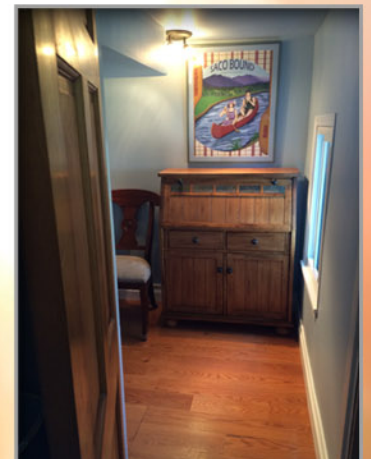
FINISHED DRYWALL PAINTED AND NEW HARDWOOD FLOOR
